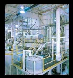
Operating a campus that includes seven battery manufacturing plants, a lead smelter, and an oxide manufacturing mill while discharging no untreated wastewater requires both a commitment to sustainable practices and sophisticated, innovative engineering. East Penn treats and reuses wastewater from its manufacturing processes in an ultramodern wastewater distillation and treatment plant that is unique within the industry.
