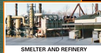
SMELTER AND REFINERY
