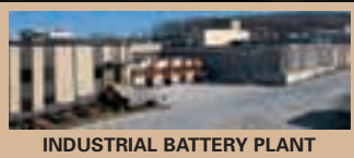
INDUSTRIAL BATTERY PLANT
